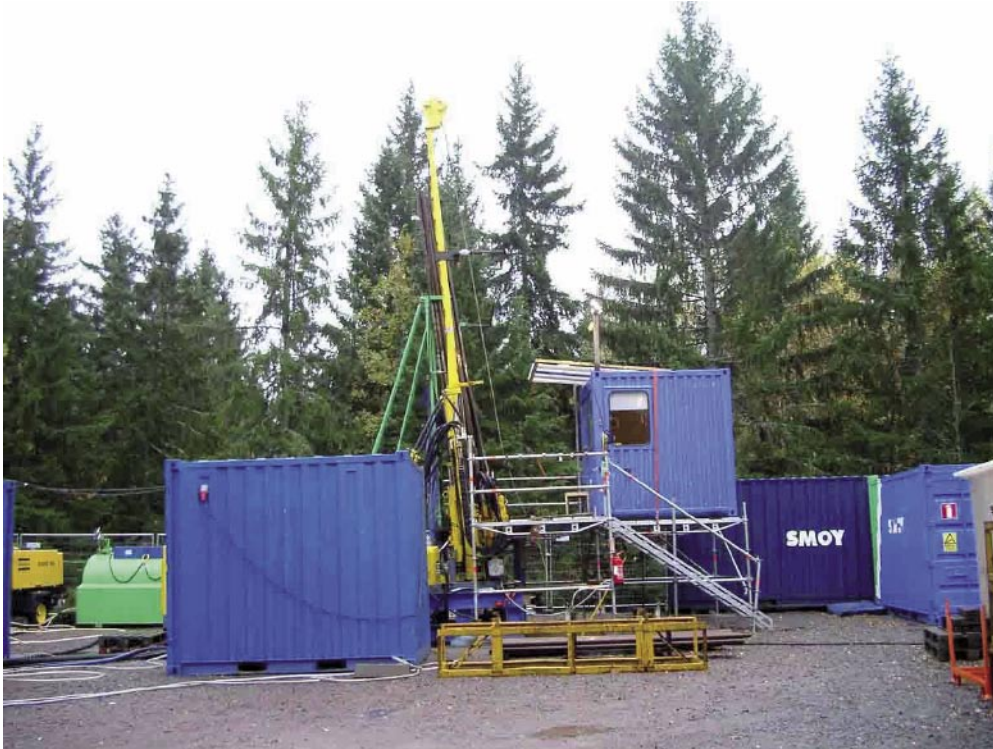
Figure 4-2. The drill site and core drilling equipment at KLX10.
