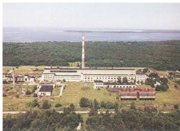
Figure 10-1. Aerial photograph of the Paldiski facility in Estonia.
