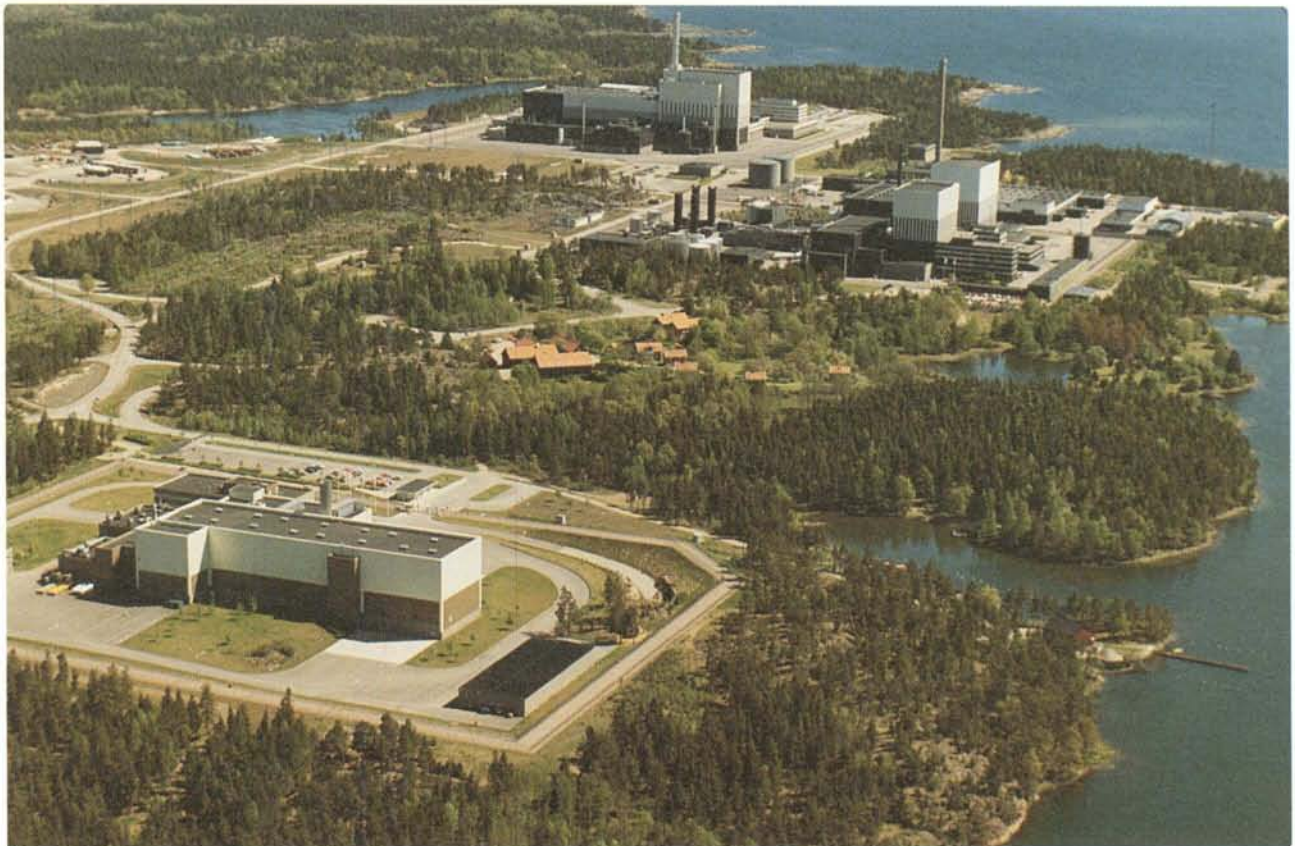
Figure 2-1. The Oskarshamn Nuclear Site. CLAB in the foreground.
