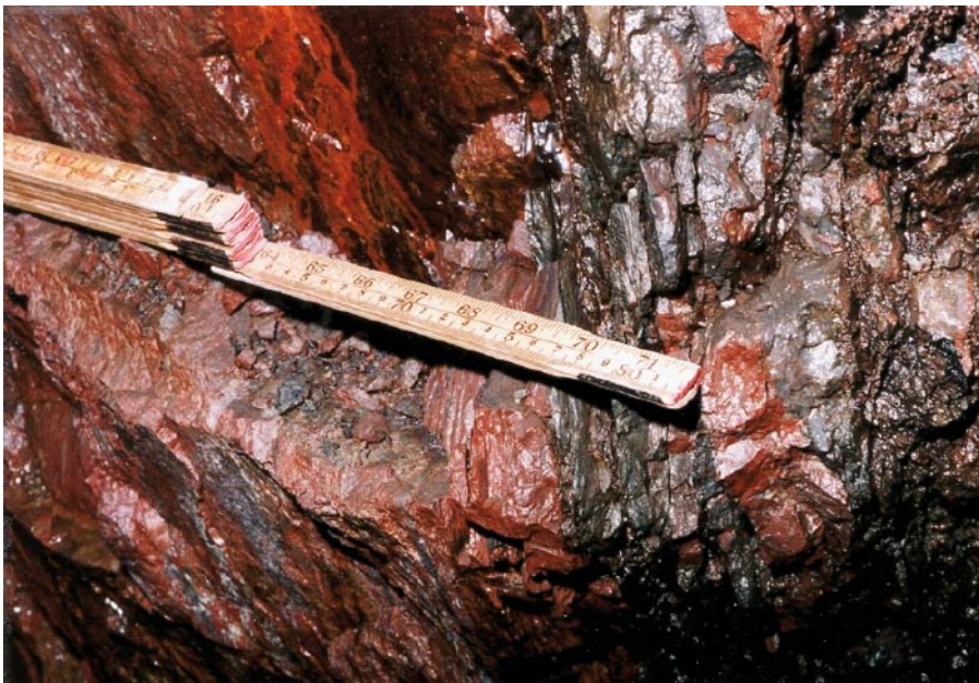
Figure 3-2. Fracture zone NE-2 at 1,605 m in the Äspö Tunnel.
