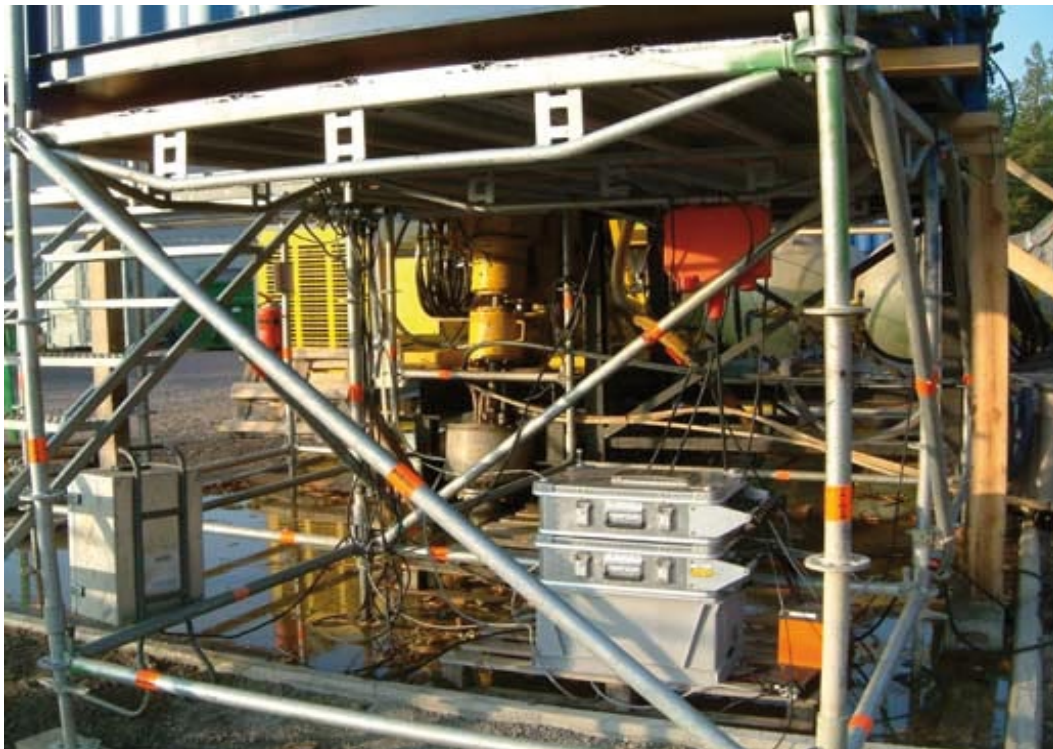
Figure 4-2. The CR23 logging unit for parameters “air-pressure” and “electrical conductivity”.
