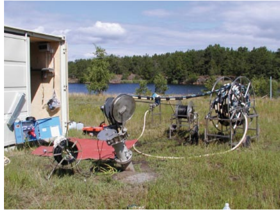
Photo 2. Equipment installed in a borehole with guiding spools on TOC.
