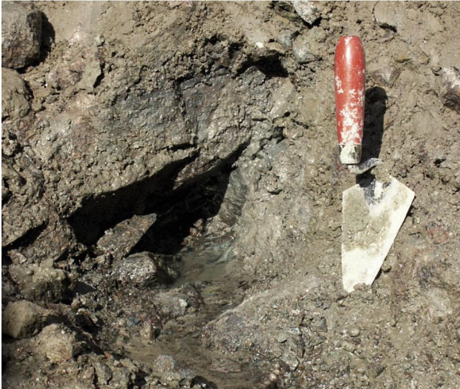
Figure 5-18. Inflow of groundwater at the transition between bedrock and Quaternary deposits, which was observed in the excavation at Profile 1.
