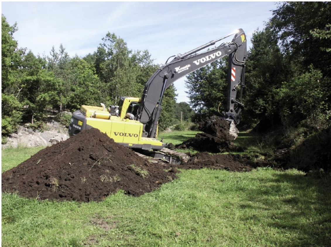
Figure 3-1. The crawler-excavator when cutting a trench at Profile 5 east of Mederhult.
