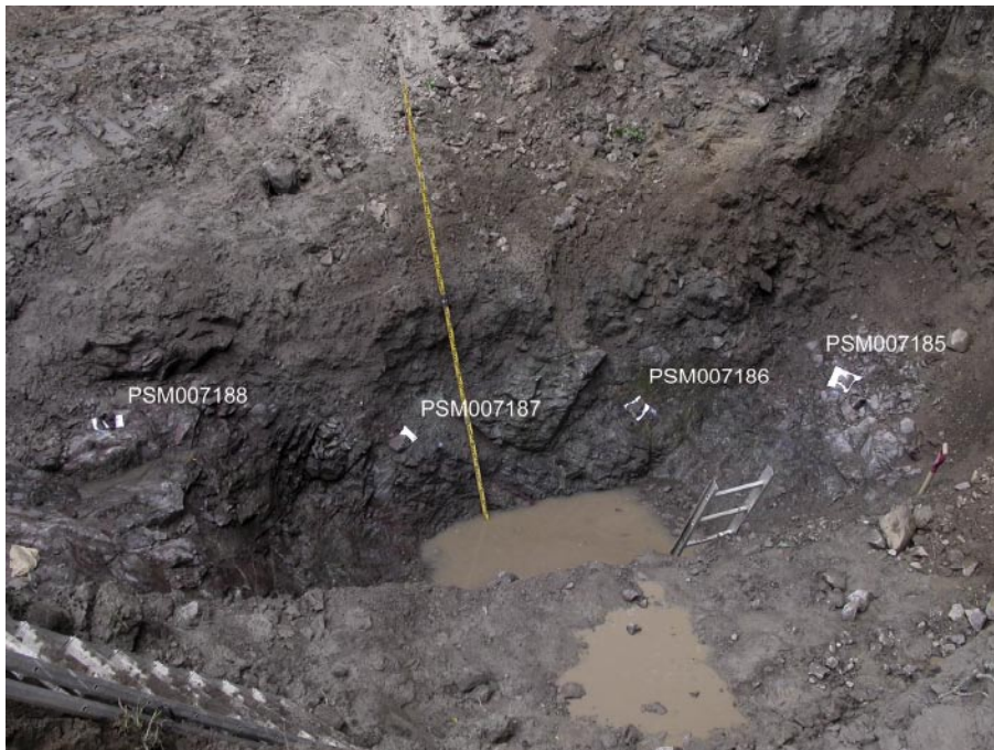
Figure 5-6. The trench at Profile 4. Looking to north-west. Observation points are marked with id-number in the picture.
