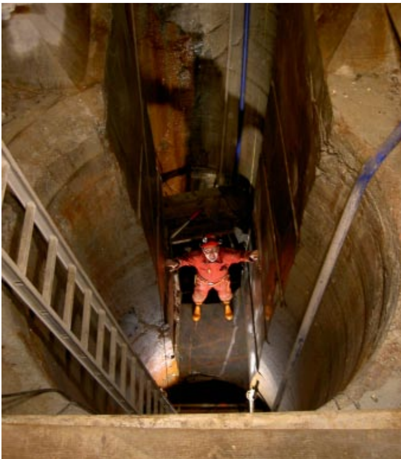
Figure 3-9. Photography of the experimental site after removal of the five one metre high pillar blocks between the two large holes.
