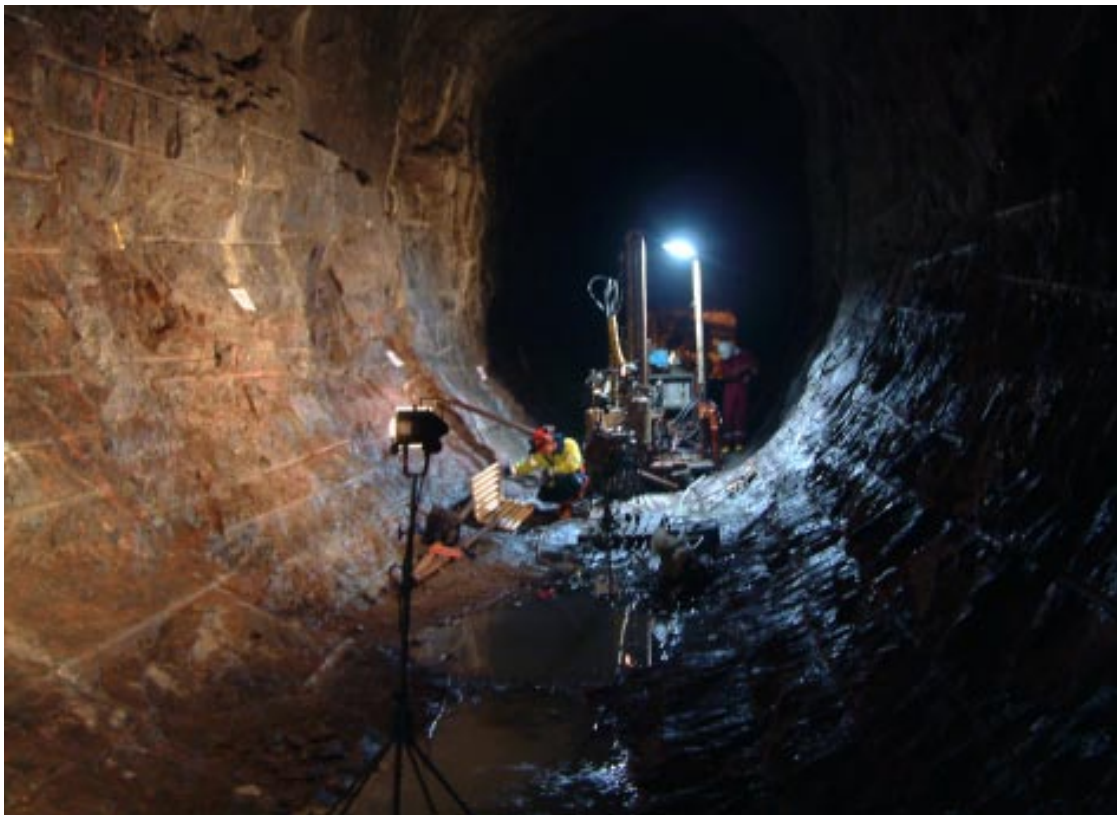
Figure 3-8. The Apse experimental drift shortly after the excavation.
