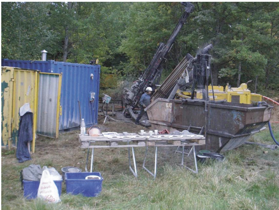
Figure 4-2. Return water from drilling (HLX37) is led to a settling container. The cyclone for collecting the cuttings can be seen fastened on top of the container. Equipment for the preliminary geological logging can be seen in the foreground.
