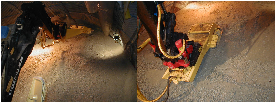
Figure 2-15. The roof compactor (left) and the slope compactor (right) during compaction.
