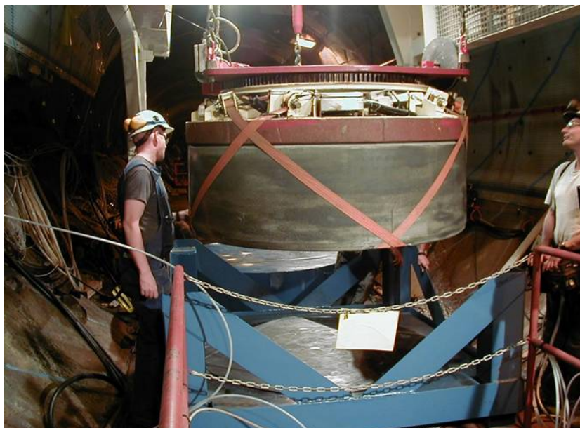
Figure 2-11. A bentonite block lifted by the four straps using the gantry-crane.
