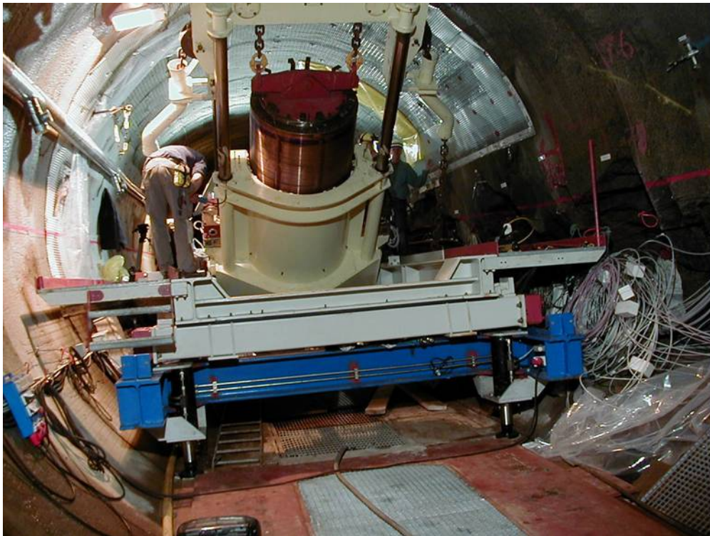
Figure 2-12. Installation of the canister with the deposition machine.
