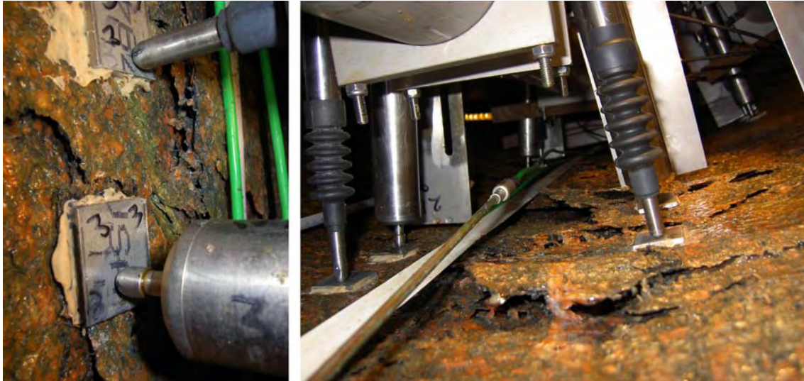
Figure 5-45. June 8. Photographs of spalling/fracturing at position #3 (2.5 m level) and between positions #9 and #10 at the 3 m level. In the right photograph position #9 is to the left.
