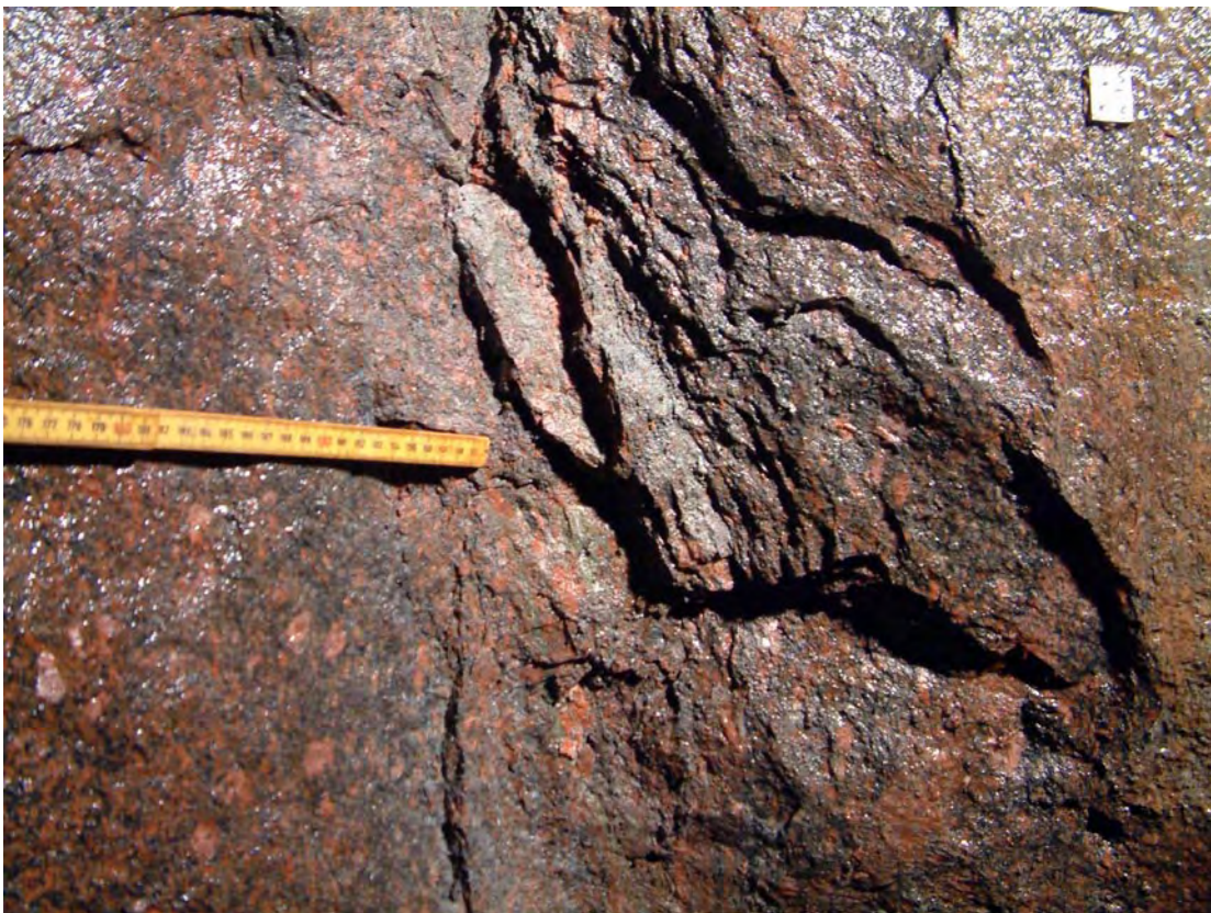
Figure 5-66. Photograph at depth of approximately 2.5 m showing the right side of the pillar, where almost no slabs could be removed.
