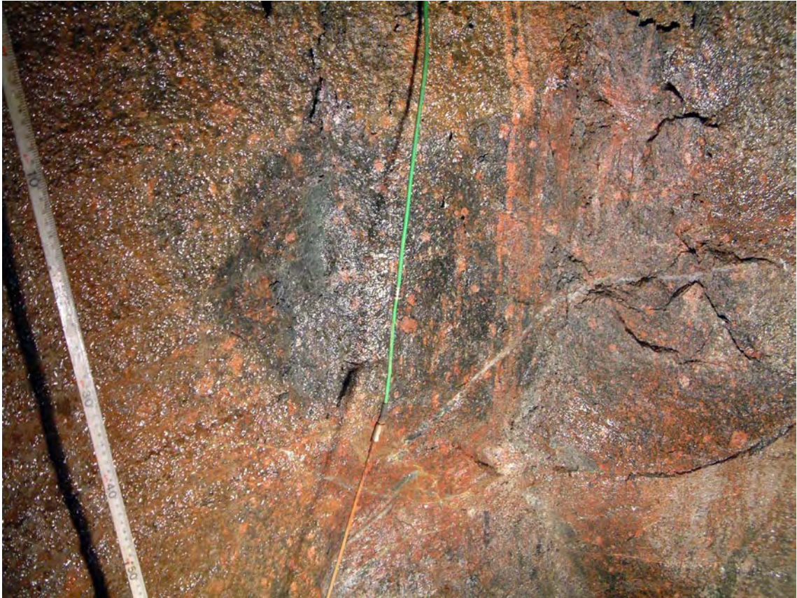
Figure 5-58. The greenstone body that created a small pit in the rock wall.
