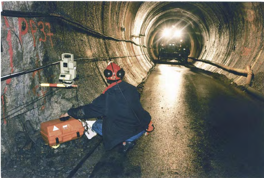
Figure 3-3. Total station mounted on a reference point in the TBM tunnel.
