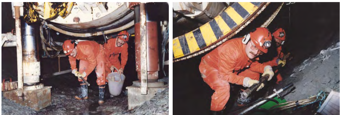
Figure 8-6. Pressure build-up tests during TBM excavation – an unpleasant activity.
