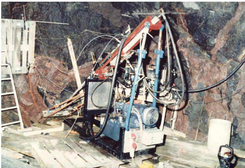
Figure 8-10. Testing equipment used for double packer testing.
