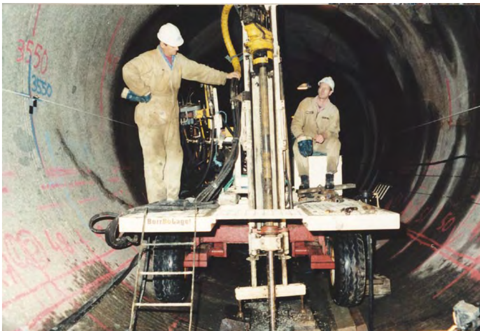
Figure 5-4. Drilling of short core boreholes in the TBM-tunnel.
