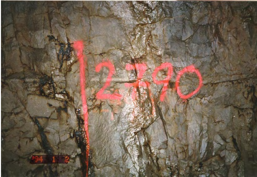
Figure 3-4. Survey line and chainage mark on tunnel wall in drill-and-blast tunnel.
