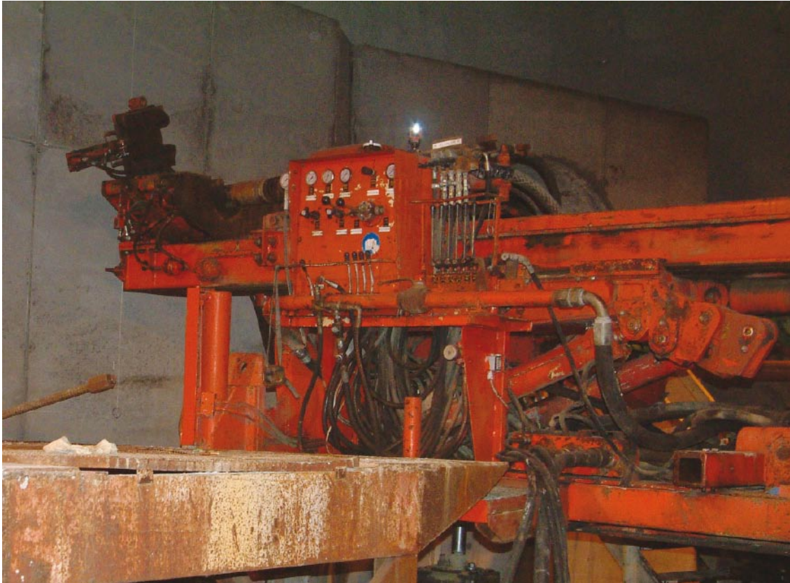
Figure 5-3. Photography of the Puntel 1200. Drilling of the 152 mm pilot hole.
