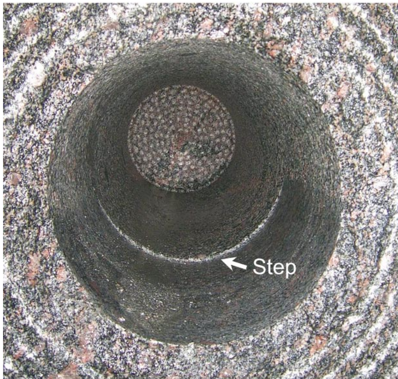
Figure 6-4. The picture shows the bottom of the 15 m pilot hole after reaming and it is evident that the guidance pin of the reamer head did not follow the pilot hole; the step is in the order of 5 mm.
