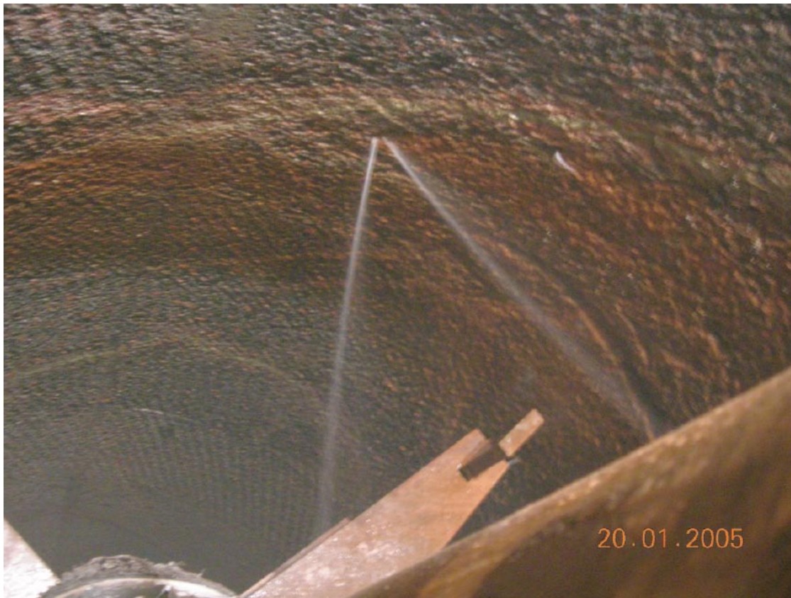
Figure 3-10. Typical seepage pattern in the drift. The inflow is channelled due to the high gradient.
