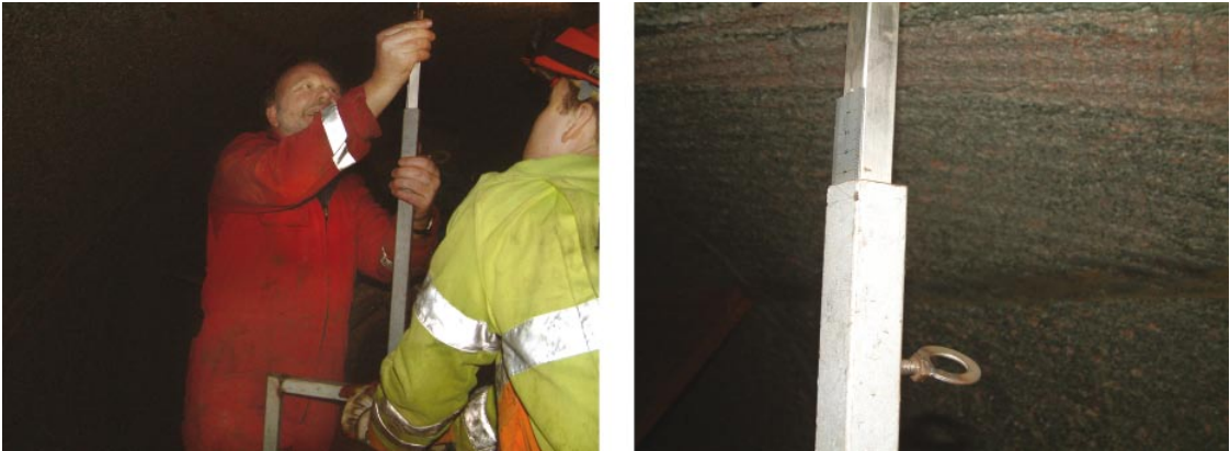
Figure 5-19. Measuring tape device for diameter measurements during reaming.
