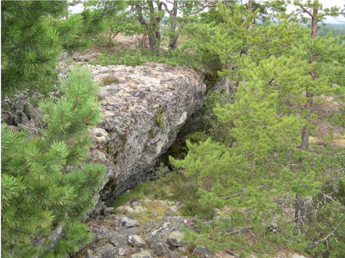
Figure 5-8. Minor escarpment along an old deformation zone at Pukens grotta. Although strongly weathered, the scarp exhibits evidence of glacial abrasion and, accordingly, is not postglacially developed.
