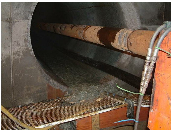
Figure 2-1 Boring of a horizontal deposition hole (KBS-3H).
