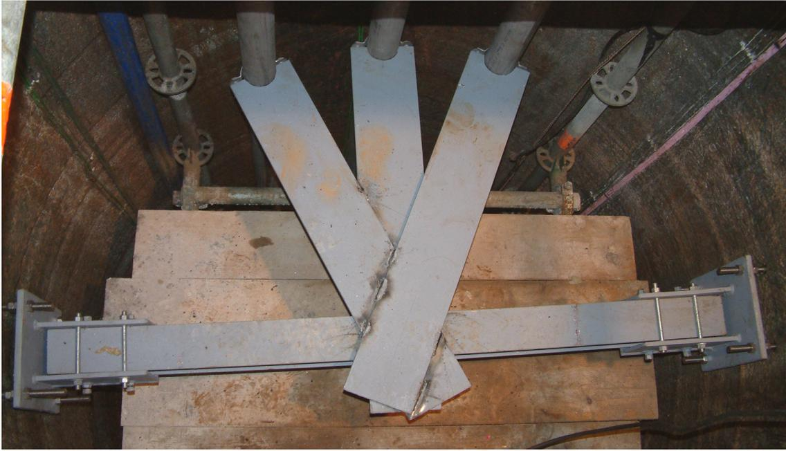
*Figure 5-8 The top mid-hole crossbar with attached plates that holds the pipes.*
