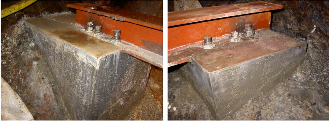
**Figure 5-5** *The top crossbar fastening. Six bolts are used on both sides to secure the crossbar.*
