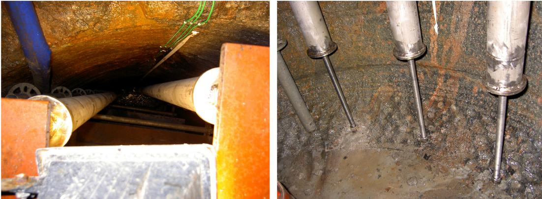
*Figure 5-1* The left image shows two of the three mounted pipes. The right image shows how the pipes are fastened to the floor in the open hole.
