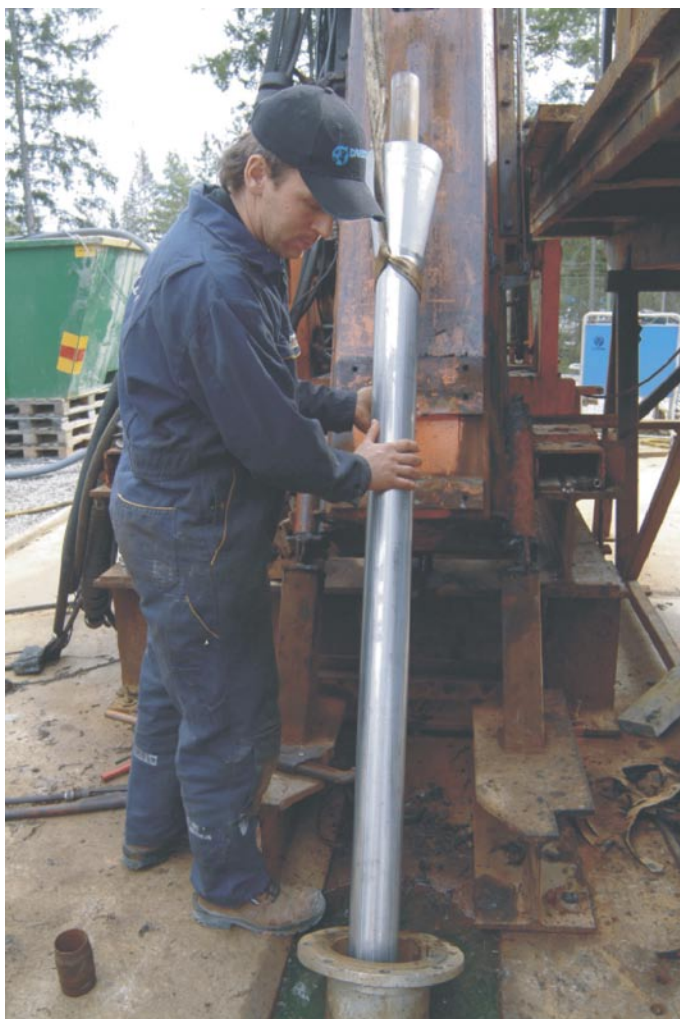
Figure 4-1. Schematic illustration of the transition cone between the upper, wide section and the lower, slim part of a telescopic borehole. In KFM07A, the entire upper, percussion drilled part was cased.
