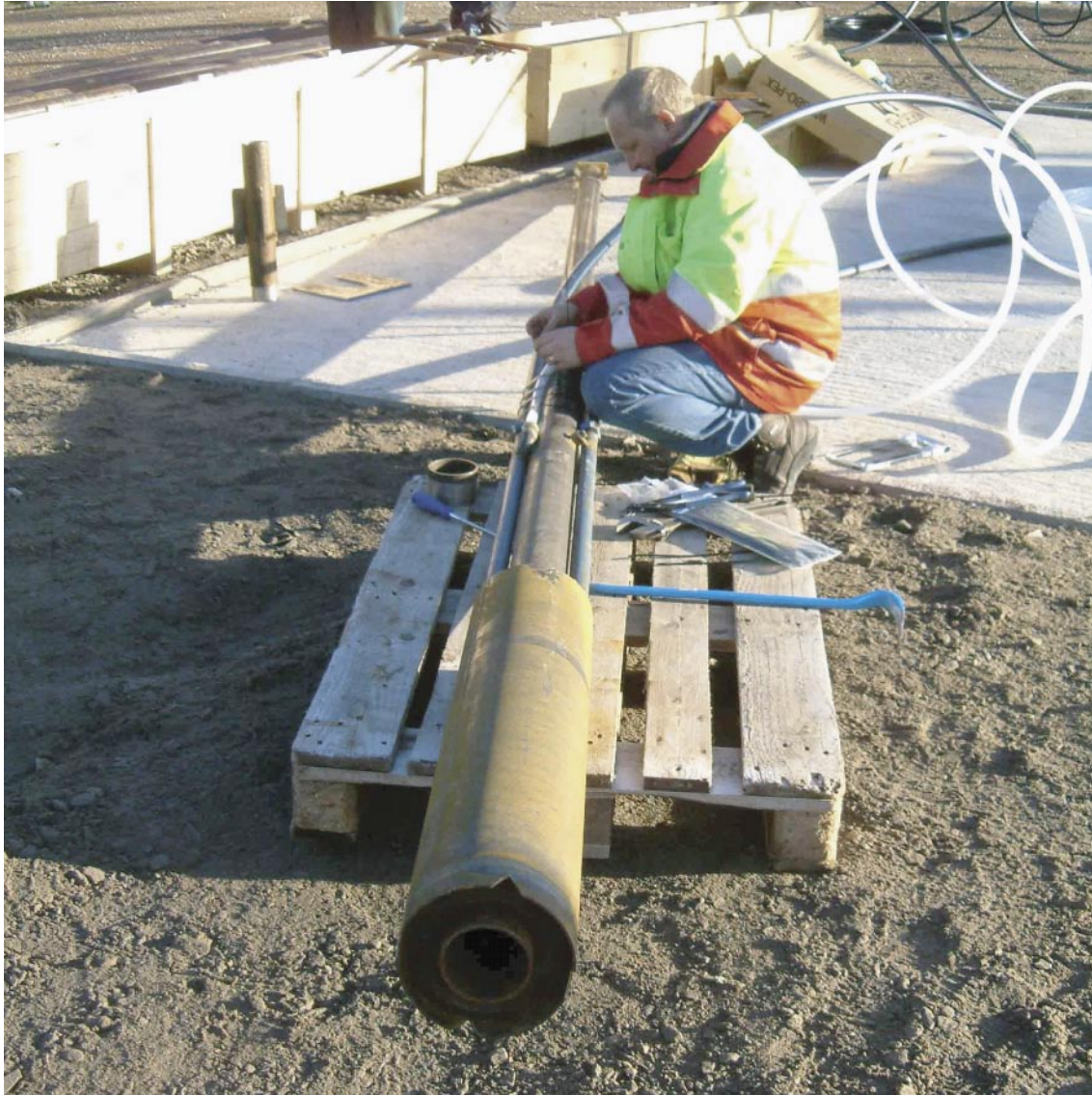
Figure 5-5. Fitting the air-lift pumping equipment before installation in the borehole.
